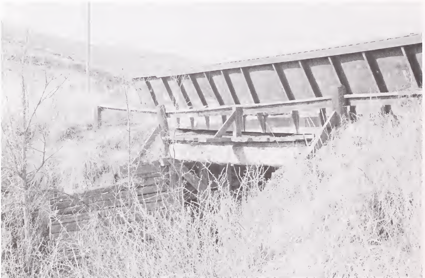
The Fourth Street Bridge in Bearcreek consists of a steel gondola railcar. It was placed on top of the remains of the timber bridge that has been located on site since at least 1914.
